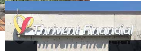
Remove Existing Channel Letters & Patch Wall
